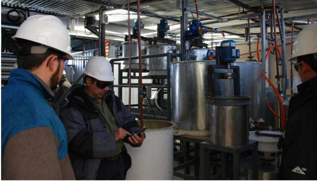
Process Development Facilities at Salar de Olaroz
