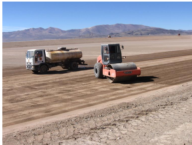
Evaporation pond 4B – Final Compaction
