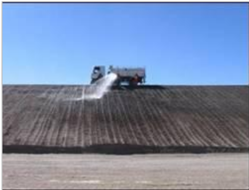
4B-evaporation pond compaction of embankments
