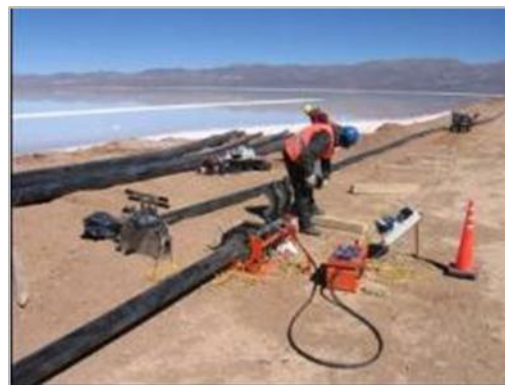
Pipe laying for brine transfer from the wells to the evaporation ponds
