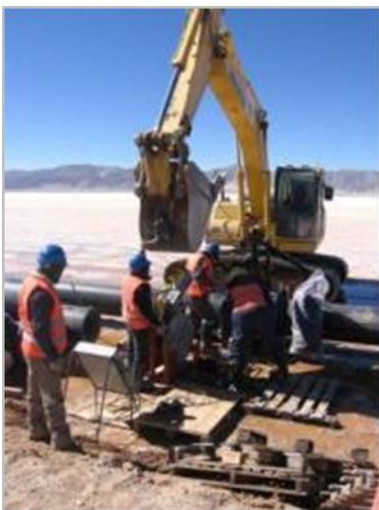
Pipe laying for brine transfer from the wells to the evaporation ponds
