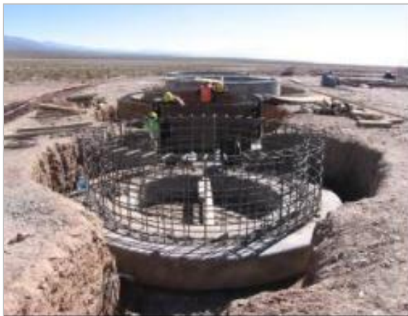
Foundation of tanks and reactors
