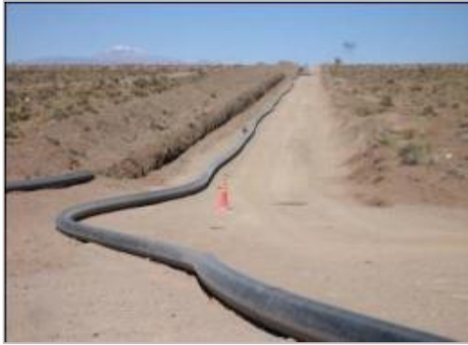
Assembly of the aqueduct pipe
