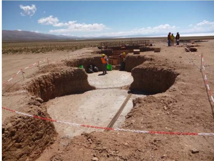
Foundations for Lime Plant Silos
