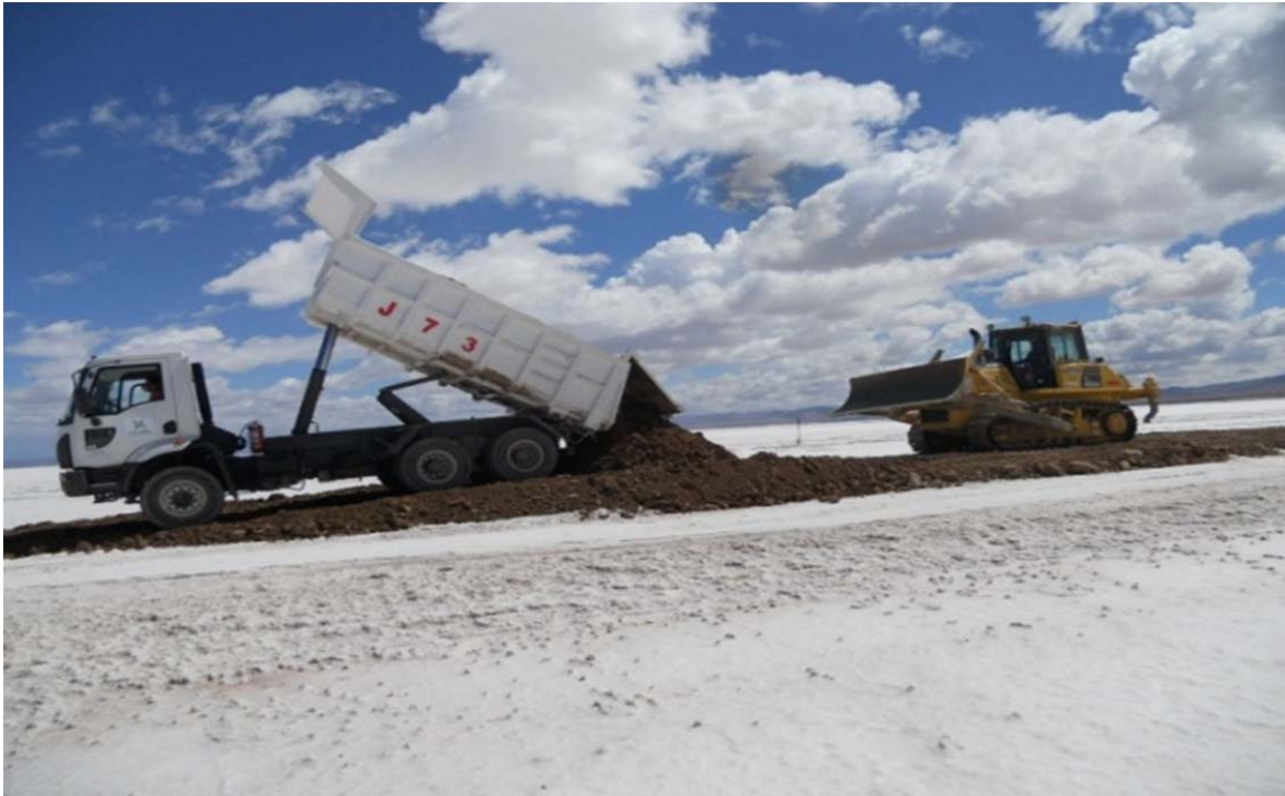
Figure 1 Building Road to Bore Field
