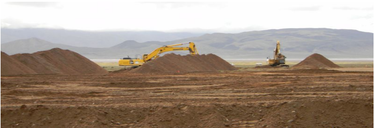
Figure 8: Construction of Evaporation ponds
