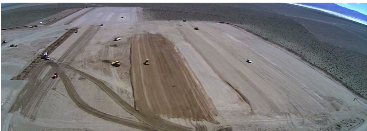
Figure 1 & 2: Aerial view of camp pad construction
