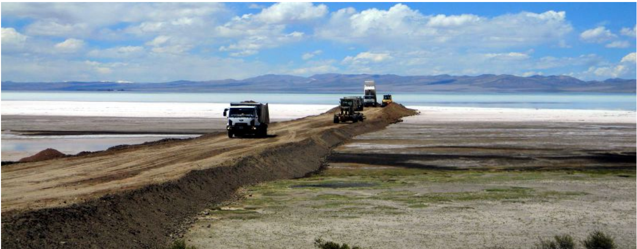
Figure 4 & 5: Construction of the main road across the salar.
