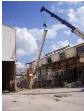
Boiler stacks being removed and loaded for relocation
