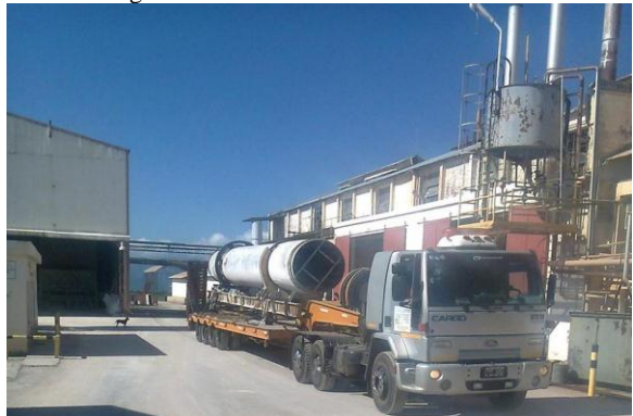
Boiler stacks being removed and loaded for relocation
