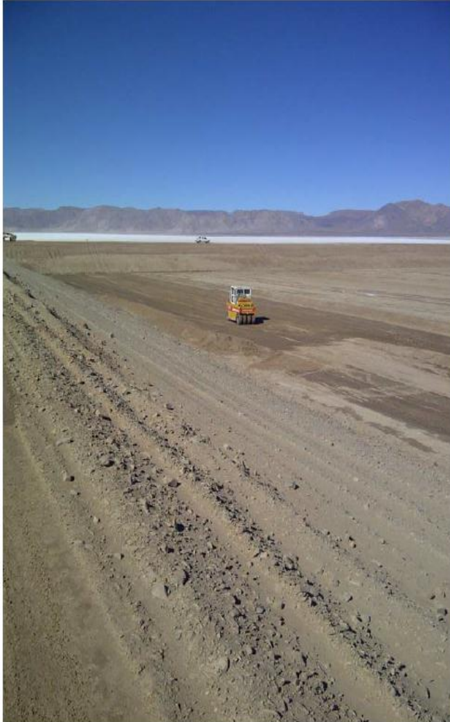
Evaporation Pond under construction
