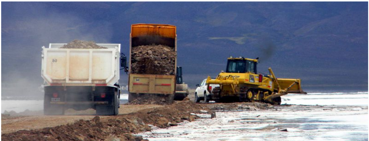
Figure 6: Construction of the road from the east side of the salar to the drilling area
