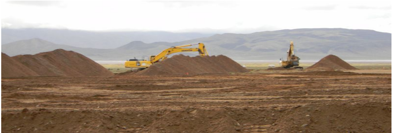
Figure 8: Construction of Evaporation ponds
